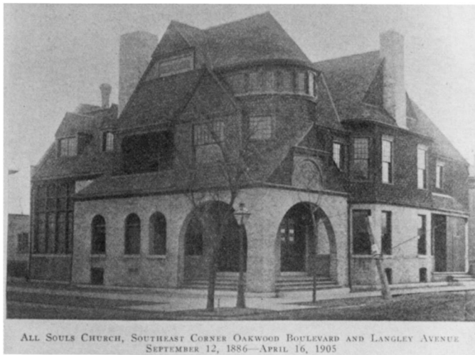
2 Silsbee, All Souls Church, Chicago, 1886, view from north-west (from Abraham Lincoln Centre [and] All Souls Church; Reports for 1912 ; courtesy Oak Park Public Library, Oak Park, Illinois)
